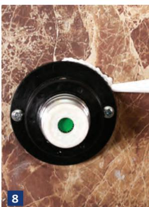
**8** Apply sealant around the fixing plates before fitting the chrome trims.
