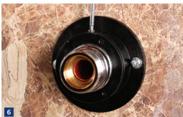
**6** Lock the fixing plates to the push-fit connectors using the supplied grub screws.
