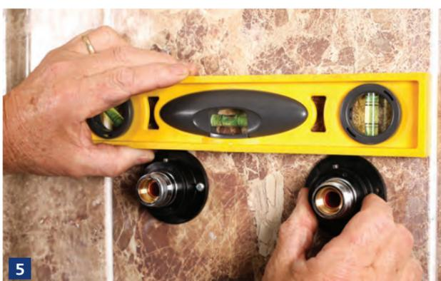
**5** Check the fixing plates are level and at 150mm centres and secure them to the wall.
