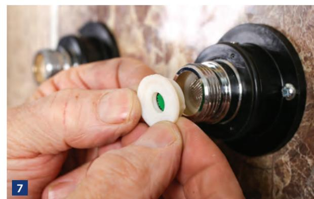
**7** Fit the filters, flow limiters if required and inlet washers. An alternative 12 l/min flow limiter is also supplied for the outlet.
