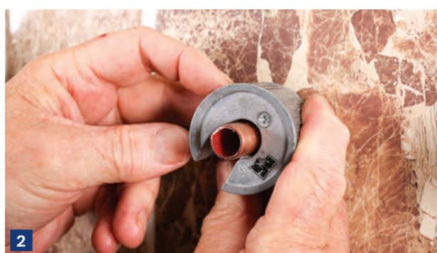
**2** Complete the supply plastic or copper pipework to the mixer bracket mounting points, leaving an excess of pipe protruding out of the wall after tiling is finished. Then cut the pipe tails to the correct length between 28 to 30mm. The supplied pipe guide tool can be used throughout the installation.
