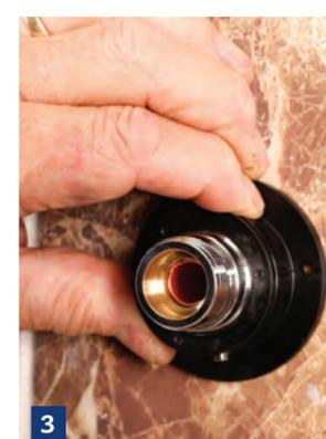
**3** Press a push-fit connector onto each pipe tail, then screw the fixing plates onto the connectors.
