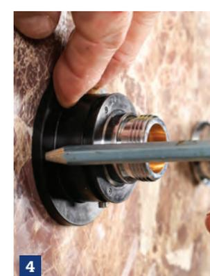
**4** Mark then drill the holes for the fixing plates – the supplied pipe guide tool can be used to hold them 150mm apart.
